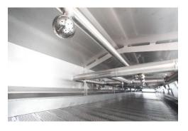
**All piping, Aisi 316 stainless steel**, is backing-gas welded. This method ensures the highest hygienic standard possible.
